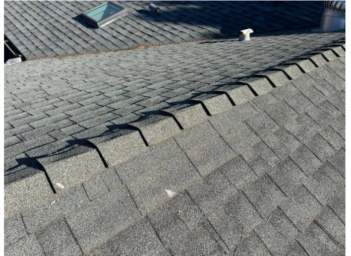
Roof photos - Roof photos
