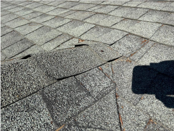
Roof photos - Roof photos
