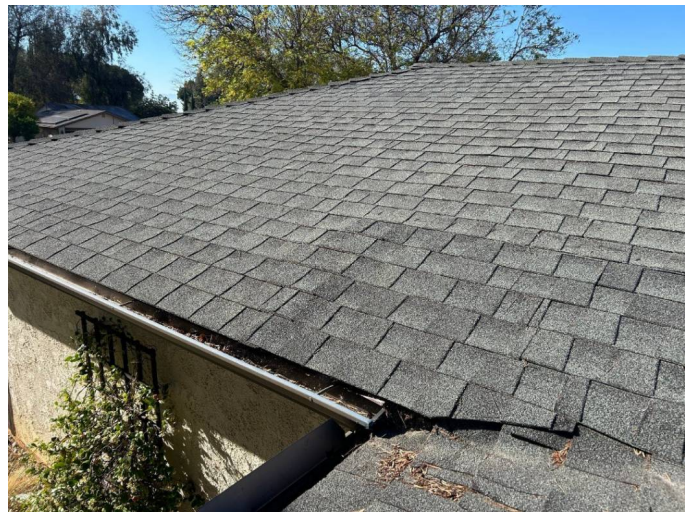
Roof photos - Roof photos
