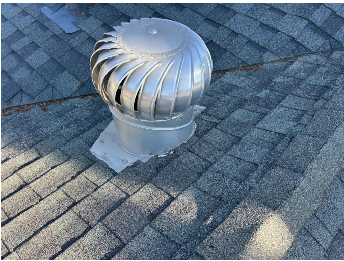
Roof photos - Roof photos
