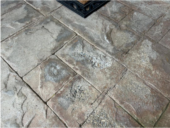
Additional photos - Additional photos
