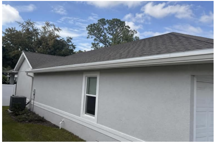
Roof photos - Left side roof slope; shingles in satisfactory condition.
