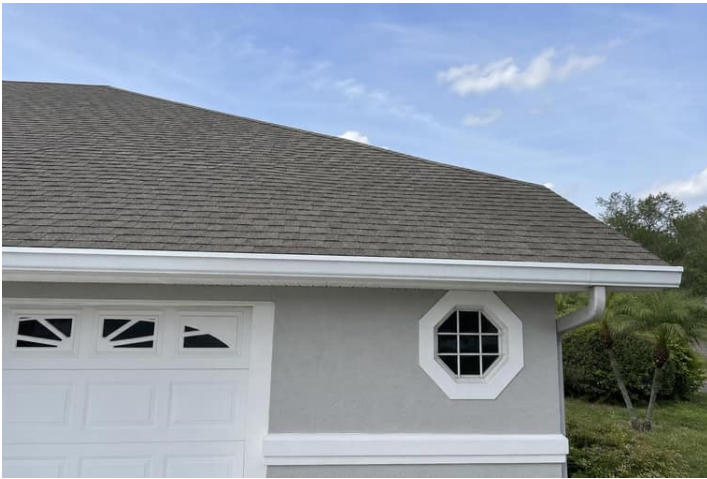
Roof photos - Front roof slope; shingles in satisfactory condition.
