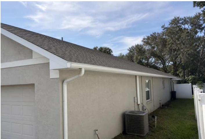
Roof photos - Right side roof slope; shingles in satisfactory condition.
