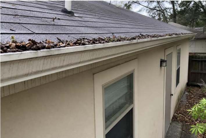
Roof 2.1a - Roof drainage and covering viewed for moisture intrusion concerns.
