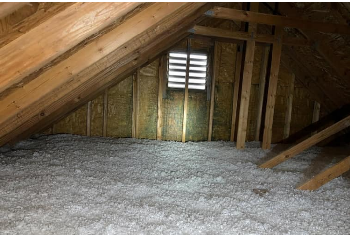
Attic, Ventilation, and Insulation 7.1a - Attic insulation and ventilation reviewed for moisture-related conditions.
