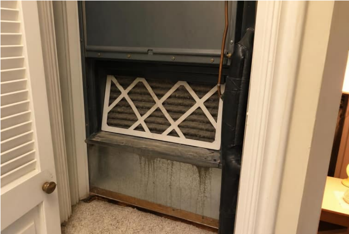
HVAC and Ventilation 5.1a - Air handler and filter area reviewed for moisture and growth indicators.
