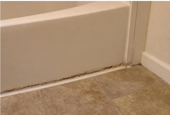
Plumbing 6.2a - Bathroom fixture and nearby finish checked for moisture indicators.
