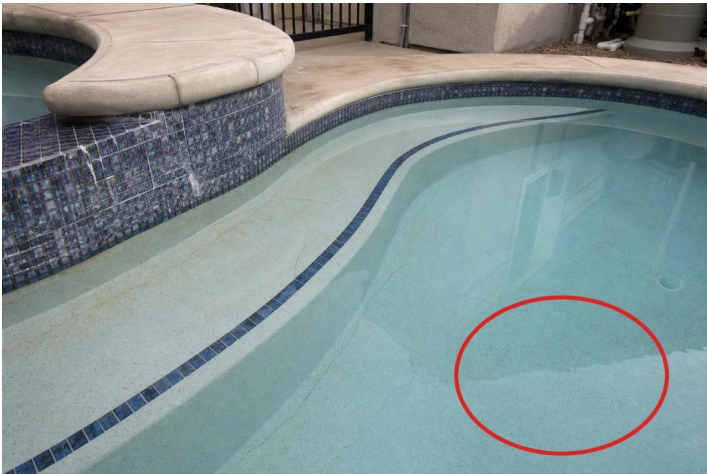
Pool / Spa Structure 1.1a - Pool/spa shell and visible surfaces
