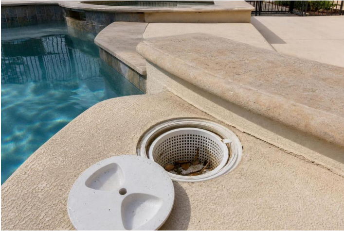
Drains, Covers, and Returns 4.2a - Skimmer weirs, baskets, and deck covers
