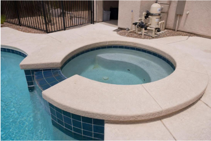
Spa Systems and Limitations 10.1a - Spa visible condition and operation
