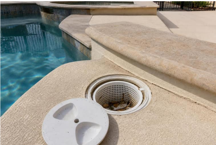
Drains, Covers, and Returns 4.2a - Skimmer basket and visible skimmer condition.
