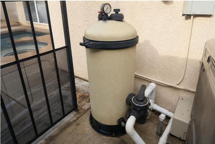
Pump, Filtration, and Plumbing 6.2a - Filter tank, gauge, and visible fittings.
