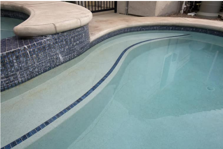
Pool / Spa Structure 1.1a - Pool shell and visible interior surface overview.
