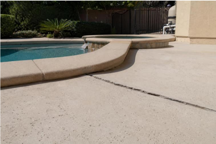
Deck and Access 2.1a - Pool deck walking surface and drainage area.
