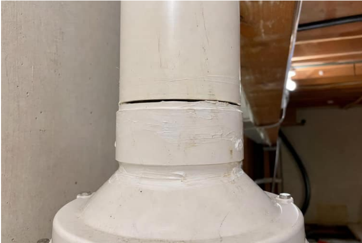
Vent Piping, Fittings, And Supports 4.2a - Accessible pipe joint with visible sealant gap.
