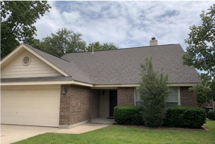
Front roof slope viewed from a safe ground-level vantage.
