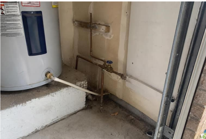
Main water supply valve and visible supply piping documentation.
