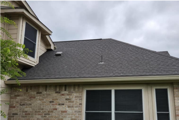
Composition shingle roof covering viewed from accessible ground and eave areas.
