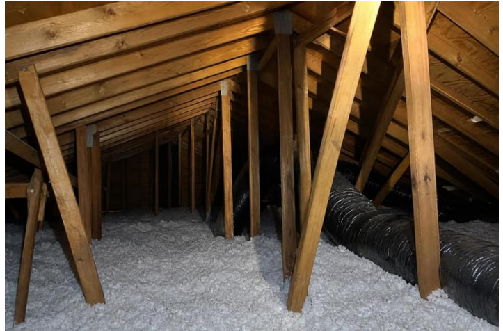
Accessible attic framing and roof decking from the attic access.
