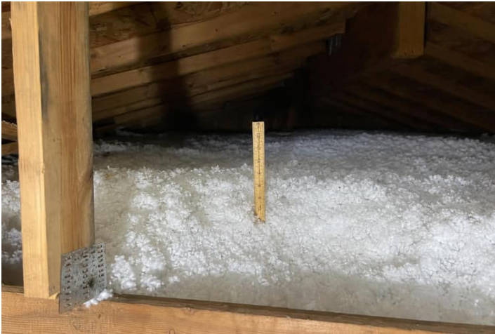
Accessible attic insulation depth documentation.
