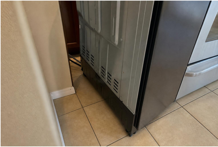
Range anti-tip bracket was not verified. - Range anti-tip bracket was not verified.
