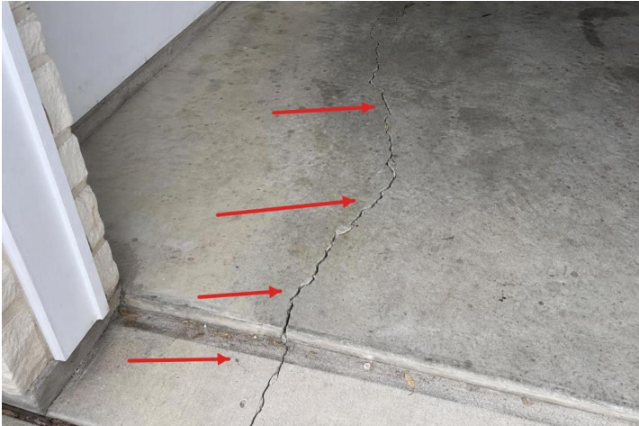
Basement, Foundation, Crawlspaces & Structure 3.7a - Foundation movement indicators
