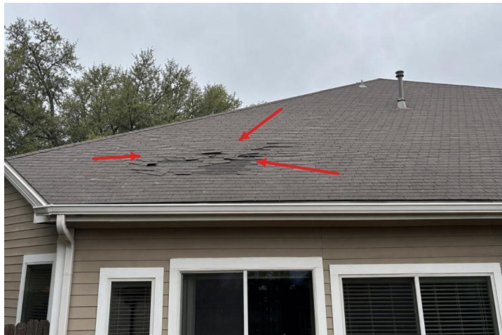
Roof 1.1b - Roof-covering materials
