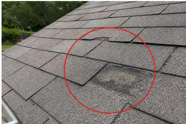
Roof 1.1a - Roof-covering materials
