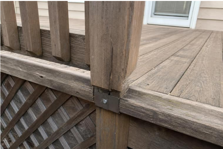
Exterior 2.8b - Closer view of guardrail post movement at the rear deck.
