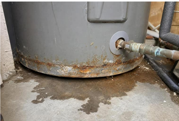
Plumbing 6.3a - Water heater corrosion visible near the lower jacket and connections.
