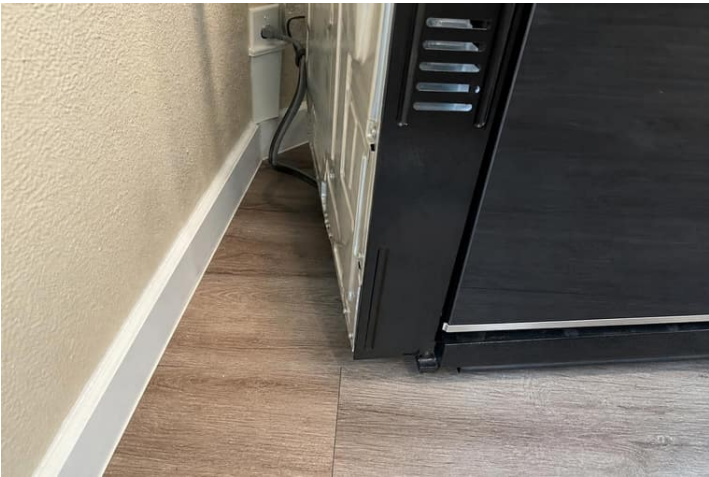
Optional Systems & Components 11.2a - Range anti-tip bracket was not verified.
