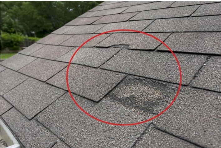
Roof 1.1a - Roof-covering materials
